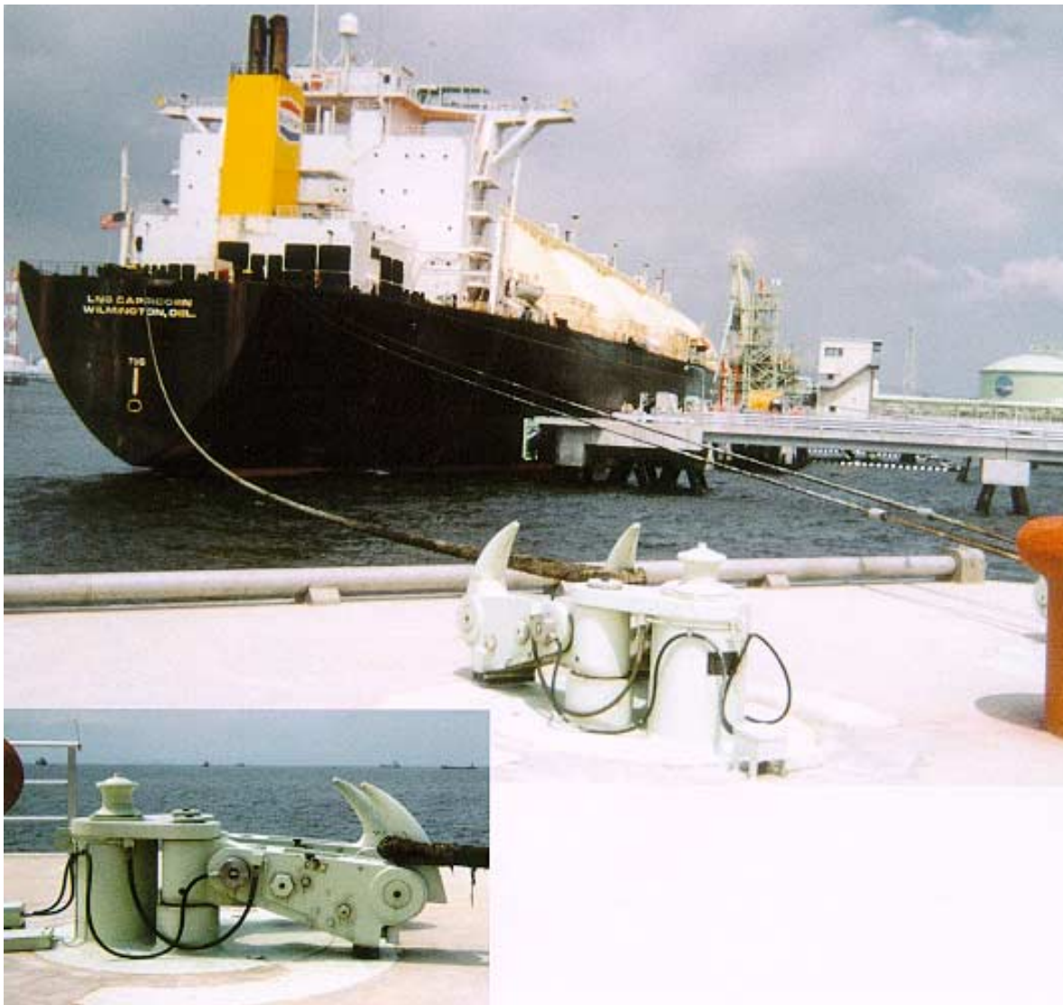
Quick Release Hook with load measuring pins fitted
